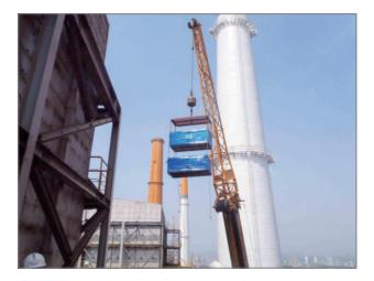
**Figure 1.** Installation of the KIST catalyst to the De  $NO_x$  system of POSCO sintering furnace.
